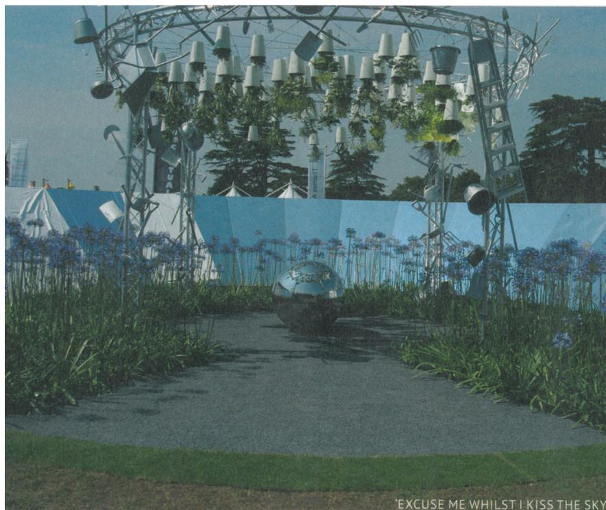
A contemporary garden designed for the RHS Hampton Court Flower Show with plants suspended from stainless steel catenary wires running between a circle of aluminium lattice struss supported on further legs of truss.
